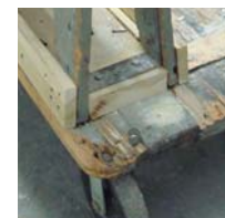
Wood—splinters and rots
